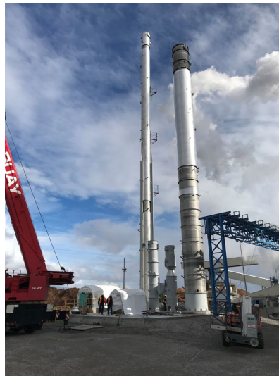
CO 2 Solutions 30 tonne-CO 2 per day carbon capture unit under construction in Saint-Félicien, Québec.
